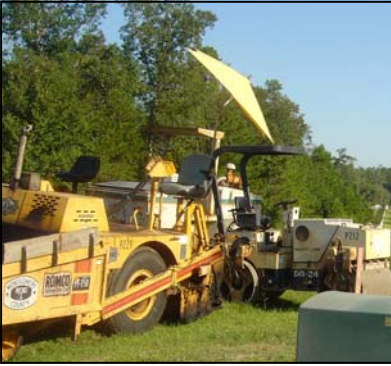
County work crew on Stone Oak Dr.
